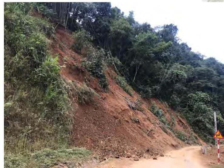
Shallow landslide along a road in MGC
